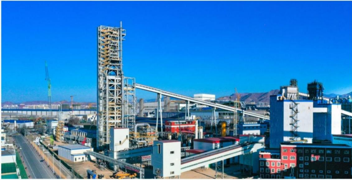
Figure 4-2-14 Hebei Iron and Steel Group Hydrogen Metallurgy Demonstration Project
